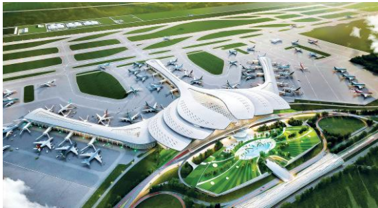
Long Thanh International Airport
