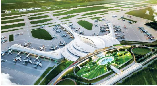
LONG THANH INTERNATIONAL AIRPORT
